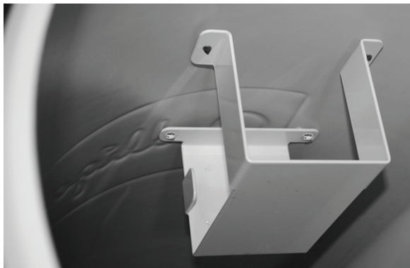
Figure 62. Softener-Cleer and solenoid brackets attached to brine tank
